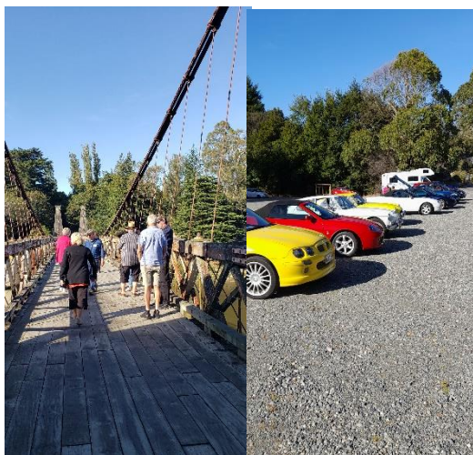
Clifton Suspension Bridge
